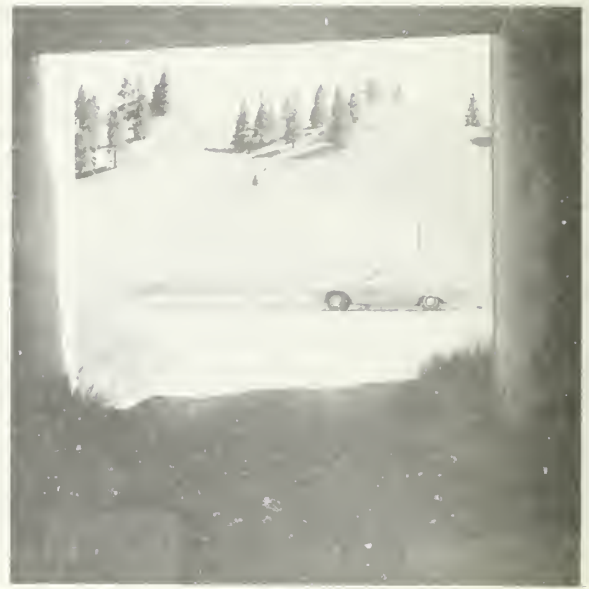
Looking north from NORTH ENTRANCE
